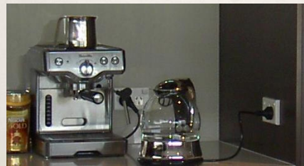
Some power points were left at the rear of bench top where known, semi-permanently placed, equipment was to go.
