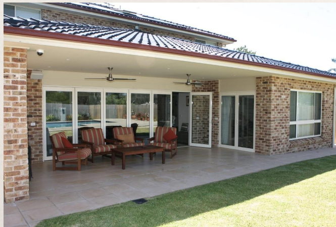
Under cover rear verandah provides weather protection to bi-fold doors.
