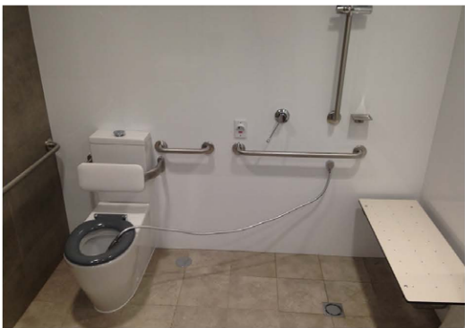
Photo 2: Disabled toilet with disabled shower head below rim of the toilet pan If reconfiguration of the plumbing fixtures does not solve the backflow issue, another solution is the installation of a proprietary fitting as shown below in photo 3. This device retracts the shower head after use and removes the cross-contamination hazard.
