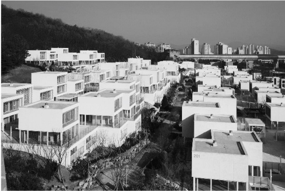
Figure 6.6 Transparent walls at Pangyo housing.
