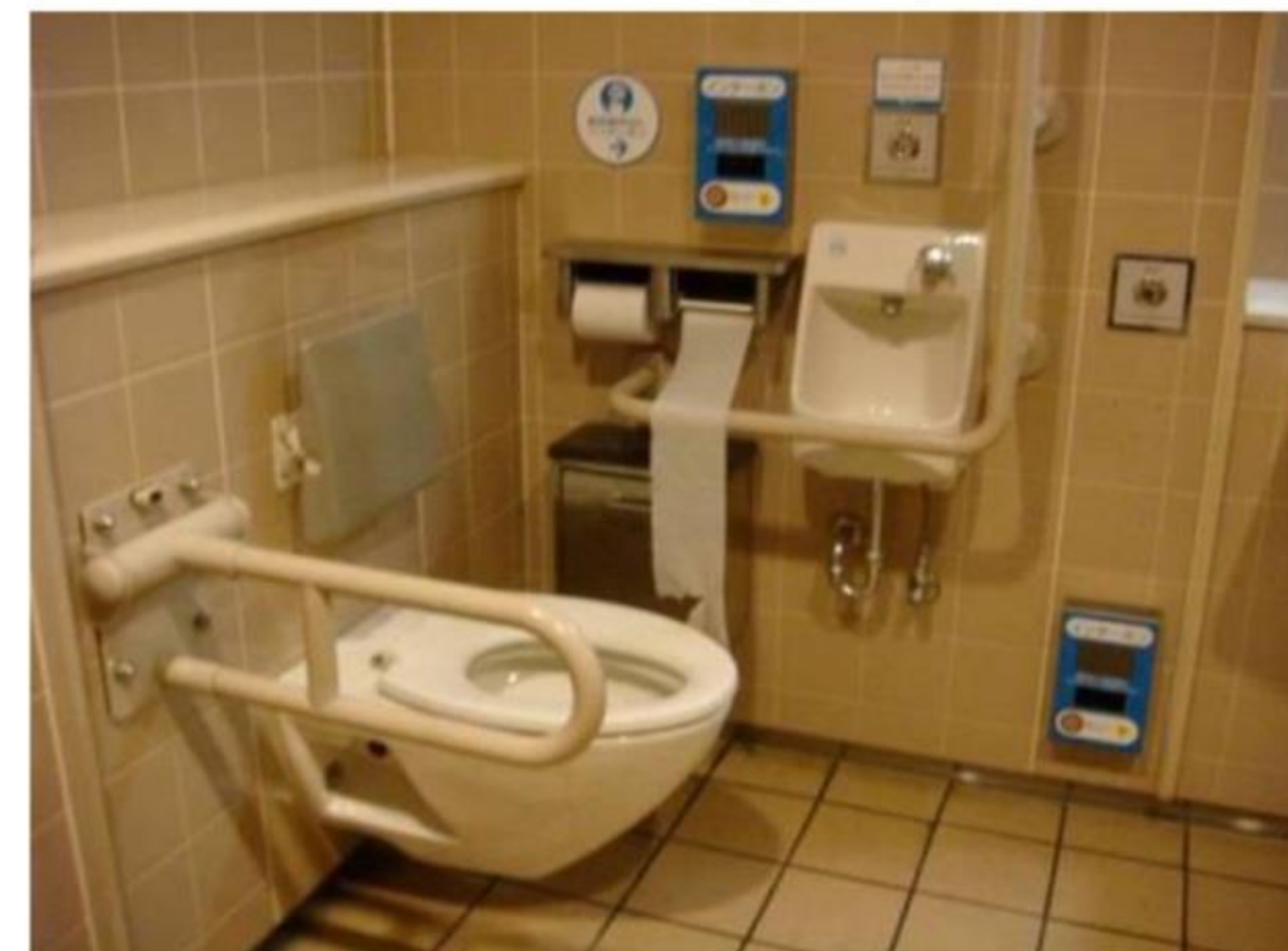
Figure 1.3: Toilet for PwDs in Japan that is fully equipped to cater for different type of disabilities (Source: NaziatyMohd Yaacob and Nor Rasidah Hashim, 2013).
