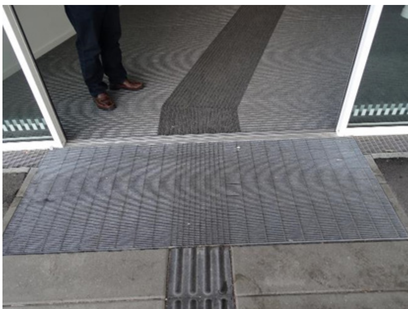
Fig 3.4b The entry to 'the most accessible office building in the world' The Disability Organisations House in Copenhagen has visual and tactile directional aids as well as a level threshold.
