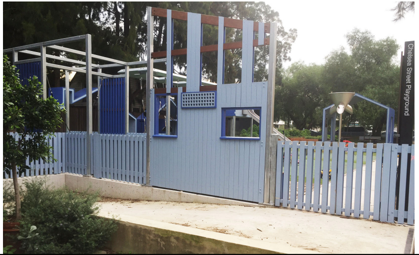
Fig 3.2a Simple step ramps are almost invisible, don't take up much space and can provide access for small, tricky changes in level.
