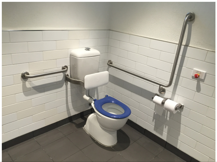
Fig 4.2a A toilet pan with a contrasting seat colour helps people with cognitive and visual impairment. Not shown here but a contrasting tiled wall behind the pan can also help.
