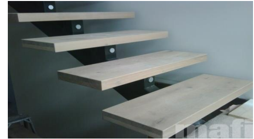
Figure 11 – Open Stair Risers
