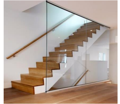
Figure 16 – Closed Stair Risers
