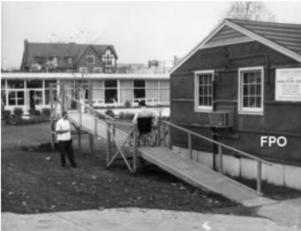
Figure 4.7. An experimental ramp for accessibility research at the University of Illinois (ca. 1950s). Courtesy of the University of Illinois Archives, image 5301.tif.
