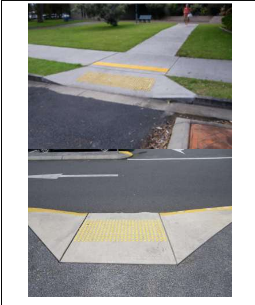
Figure 0-4: Inconsistent placement of tactile markers in the same location
