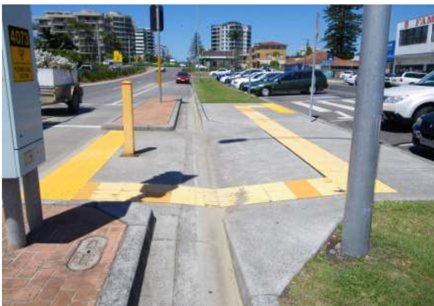
Figure 0-5: Confusing application of tactile markers
