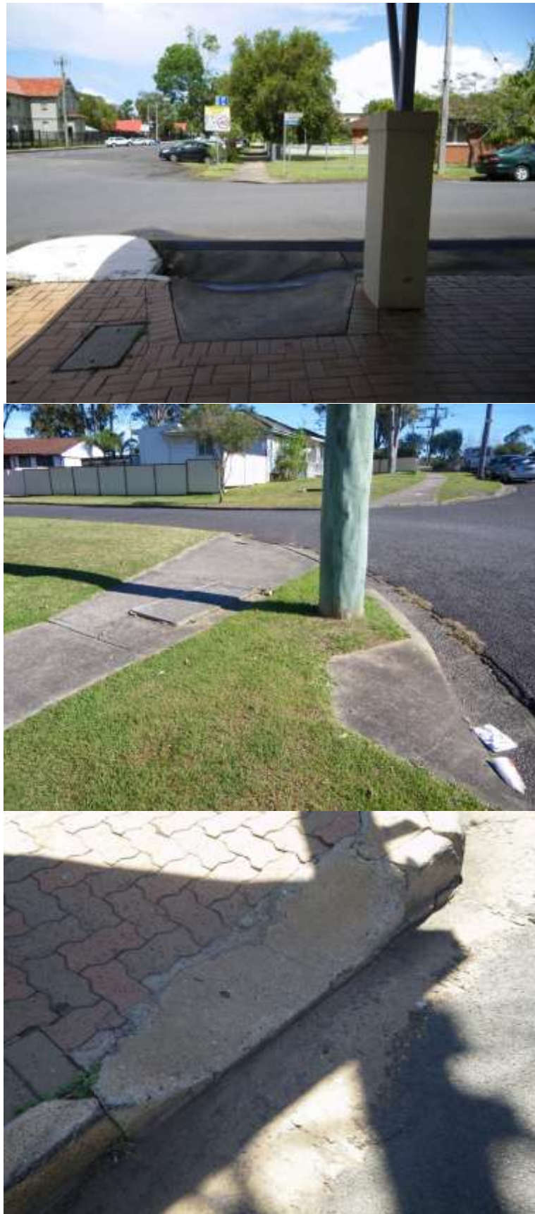
Figure 0-3: Kerb ramps poorly designed and constructed
