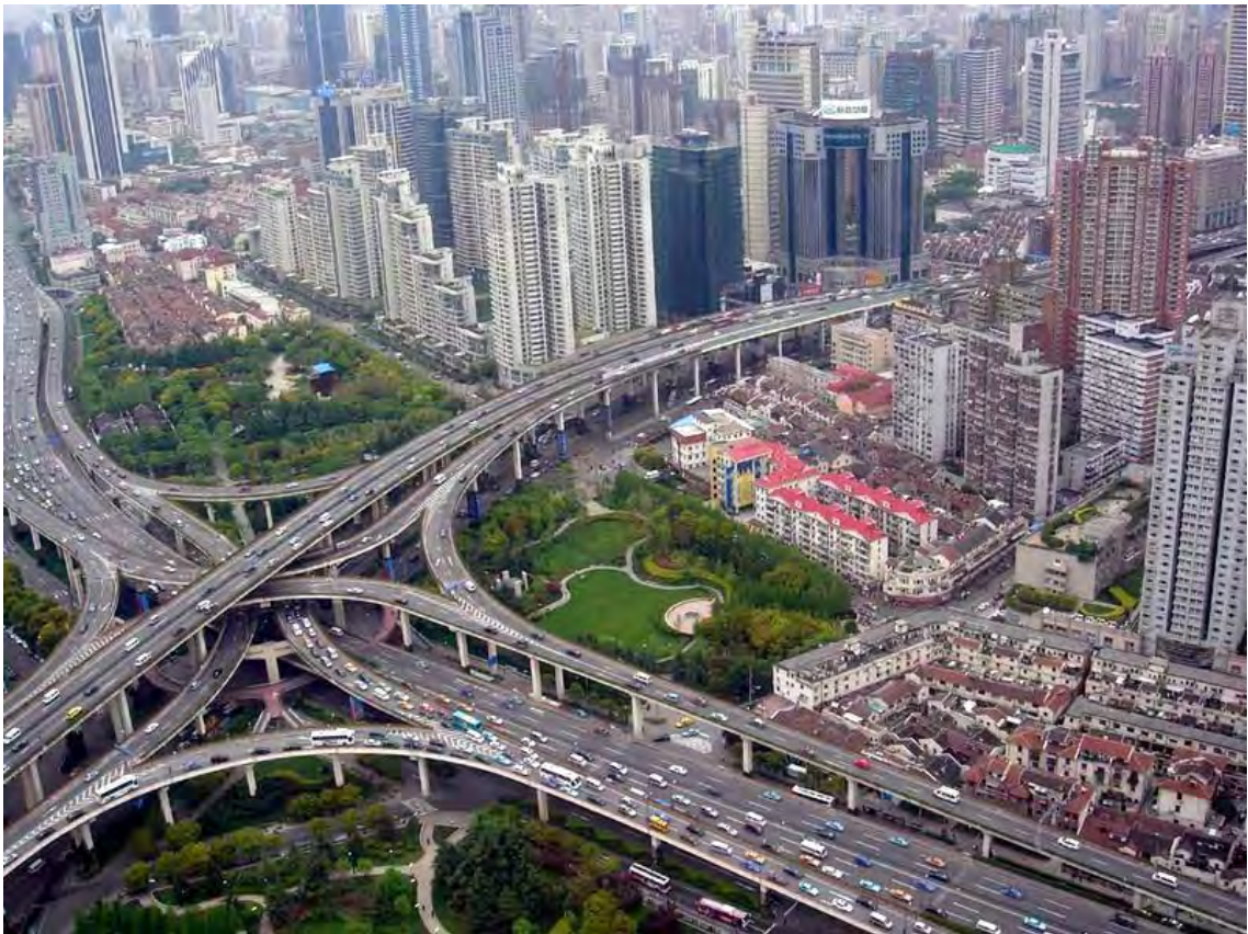
"Viaduct in Puxi, Shanghai" by Alex Needham. Licensed under public domain via Wikimedia Commons
