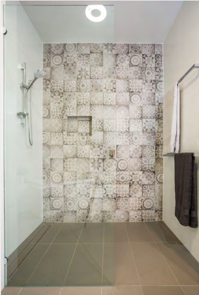
↑ In the bathroom, plan for a lip-free shower recess with screens that can be removed in future if required for easier access.
