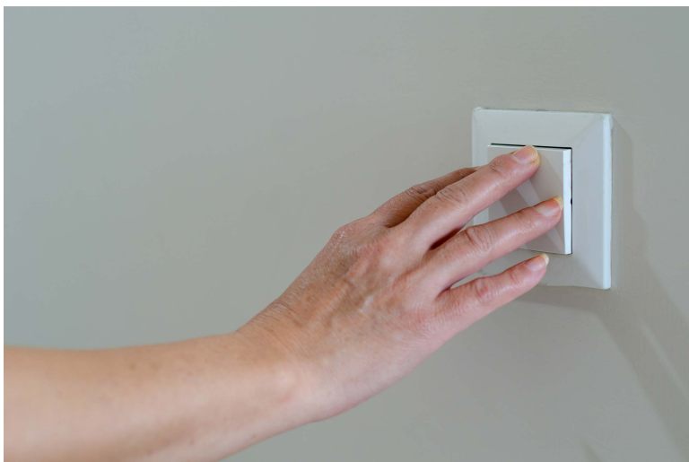
Figure 2.8 Large rocker switches for lights and power outlets allow tolerance in use.
