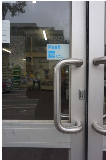
Figure 2.4 A typical 'Norman Door' where the handle suggests it should be pulled to open, so a sign is required to tell the user to push. Design for intuitive use could remove confusion. Credit: Imogen Howe
