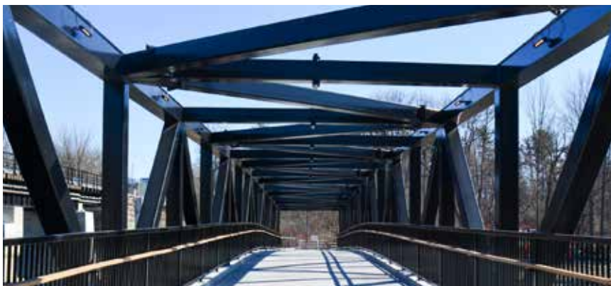
figure 48. New pedestrian bridge across the Rideau River
